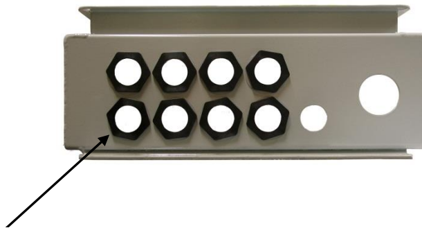
Reducing adapters shown installed
